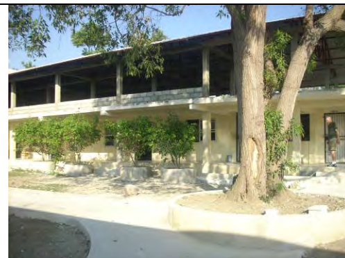
New sidewalks placed by local masons help eliminate dust and reroute foot traffic around foliage on the hospital courtyard.
