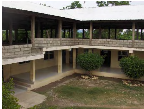
A roof has been placed over the hospital's second floor.
